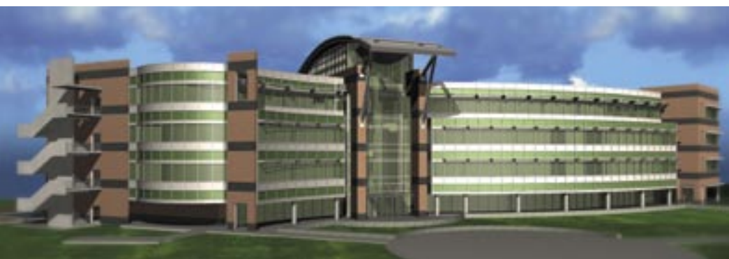
The Engineering III Building is slated to open in fall 2005.
